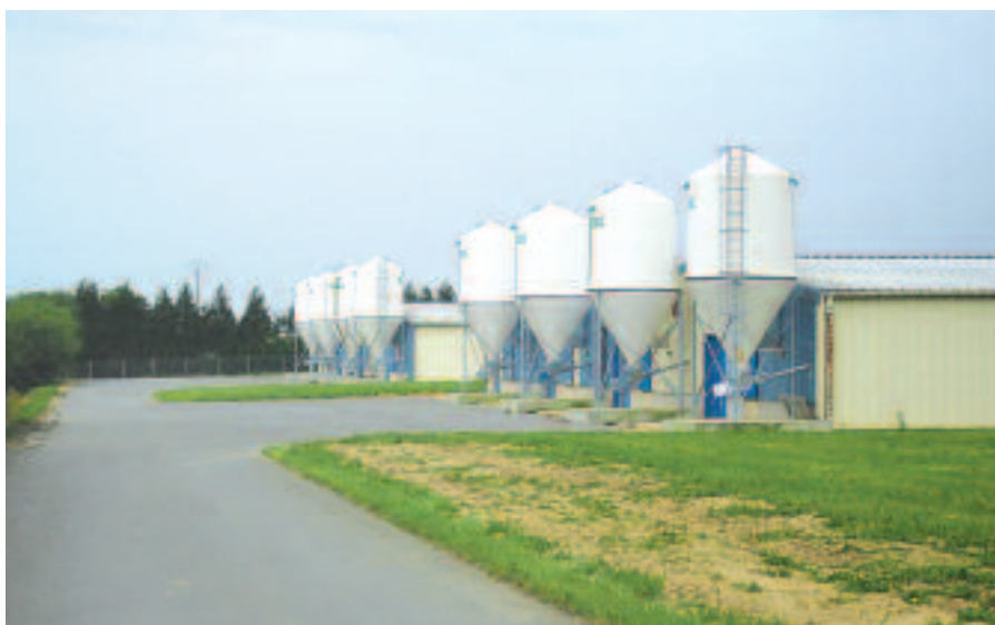
On site at Chateaubourg.
